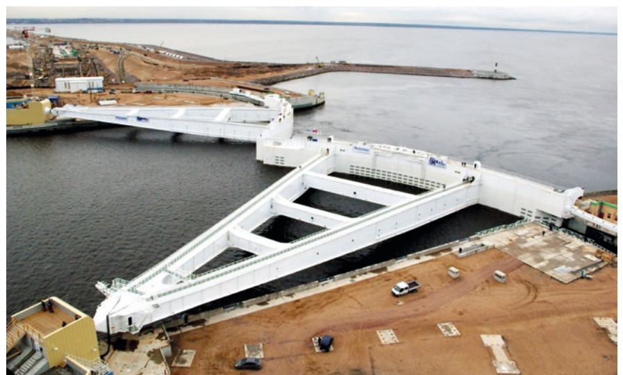
Floating gates for St. Petersburg flood protection barrier designed by Rubin is unique marine engineering facility (photo: CDB ME «Rubin»)
